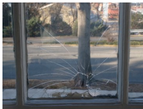
One of several panes in the master bedroom window
